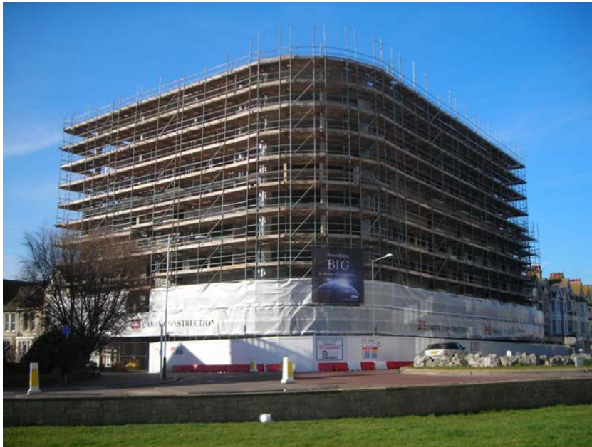
Figure 3.1 Cardy Construction Ltd. site for designer apartments in Bexhill, East Sussex.
