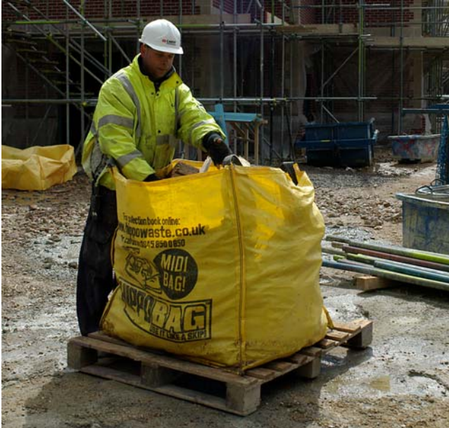
Figure 2.1 HIPPOBAGs™ being used to collect wastes on site.
