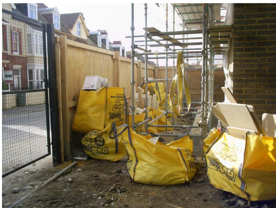
Figure 3.3 Location of waste storage area at southern side of site.
